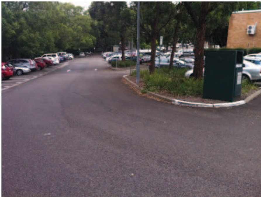
Photo 5.2.7 – Northern end of William Street roadway, looking south east
