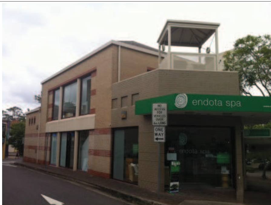
Photo 5.2.1 – Eastern end of 4 William Street, looking west
